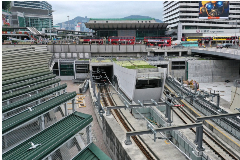
Aerial drone view of the Hung Hom MTR station on the Sha Tin-Central link. Photo: Winson Wong
